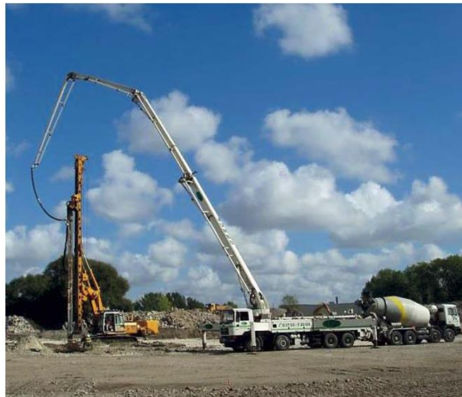
Concrete placement for VCC column
