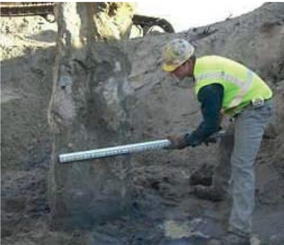
Excavated VCC column
