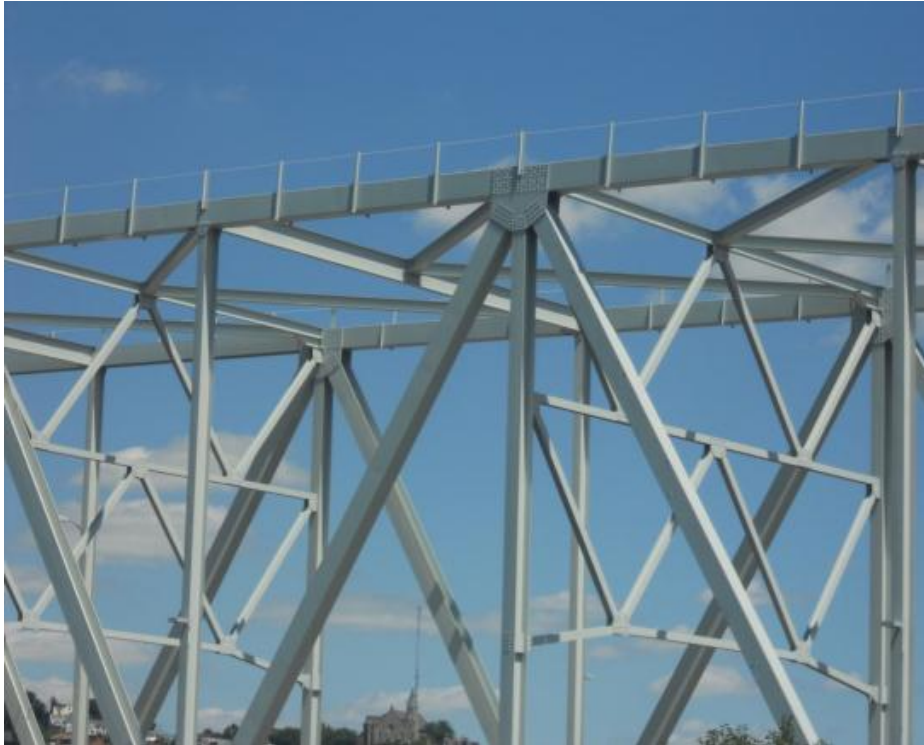
Sway Bracing and Verticals
