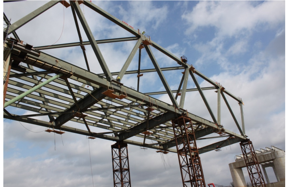
Phase Two: Superstructure and Approaches
