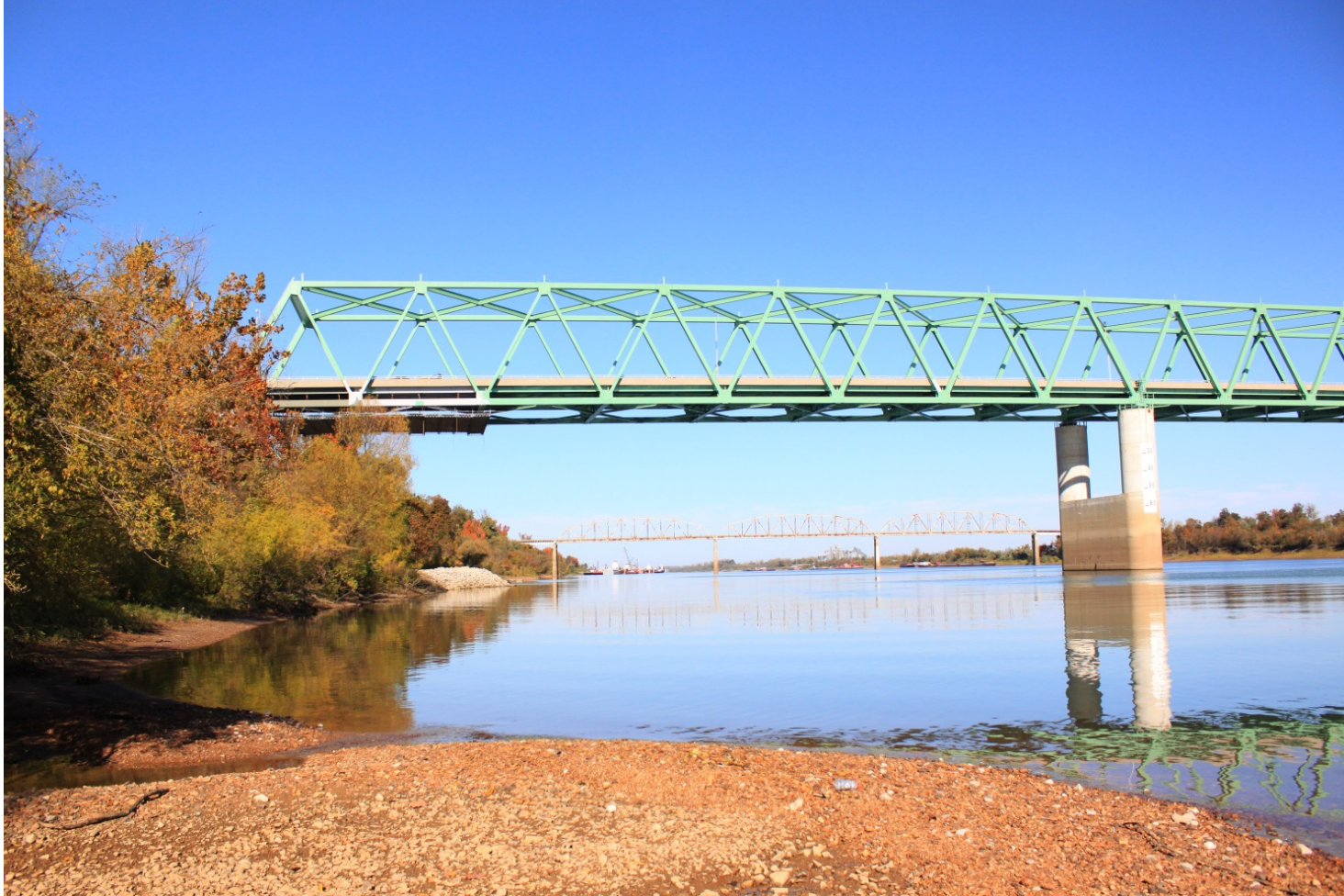
US60 Tennessee River Bridge
