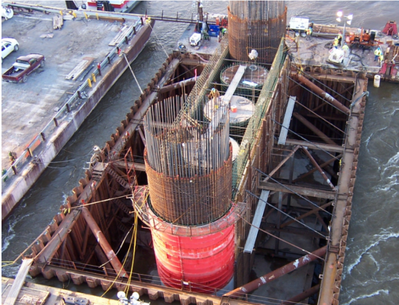
Phase one: Substructure
