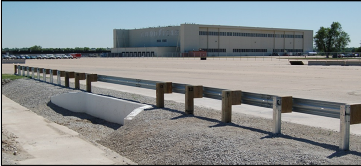
Figure 1. Midwest Guardrail System 25-ft Long-Span Design
