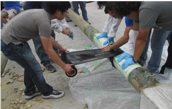
Figure 4.5: Holding GFRP sheet around the pile by Saran TM plastic wrap
