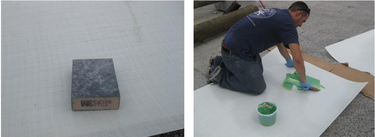
Figure 4.2: Surface roughening and application of epoxy to GFRP sheet
