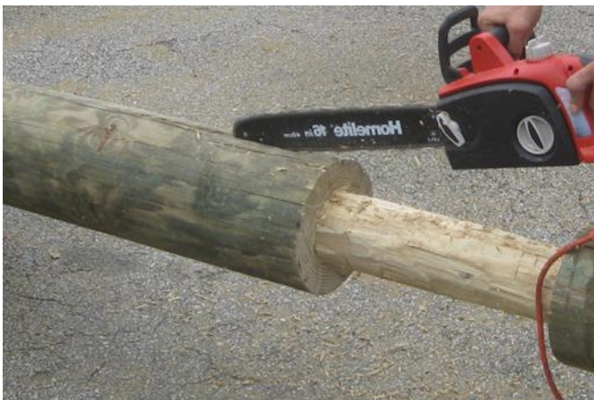
Figure 4.3: Preparing pile for GFRP sheet
