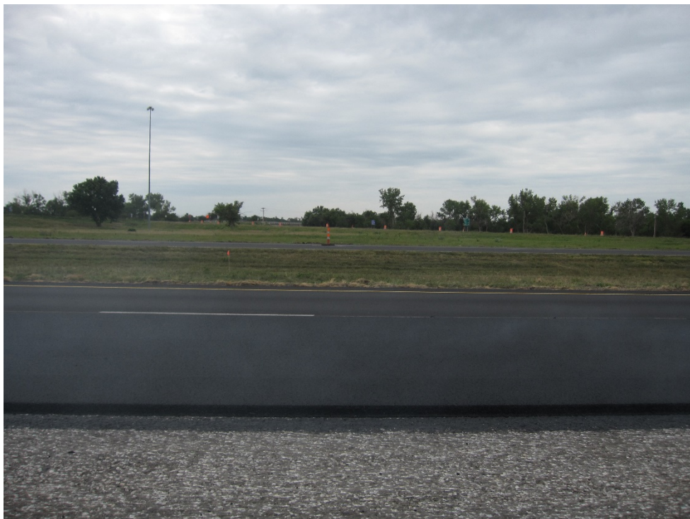
(b) new overlay paved
