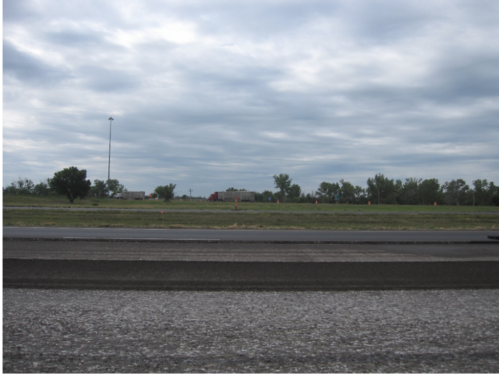
(a) old asphalt layer milled
