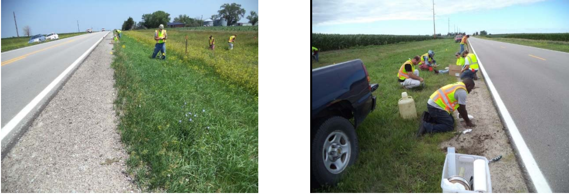
Figure 2-2. Photos taken during soil sampling at the Beaver Crossing site.
