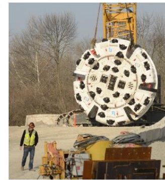
A tunnel boring machine with a 20-foot diameter cutter head is now drilling the Deep Rock Tunnel Connector, the first segment of the 25-mile Indianapolis Tunnel System that will capture combined sewer overflows.
