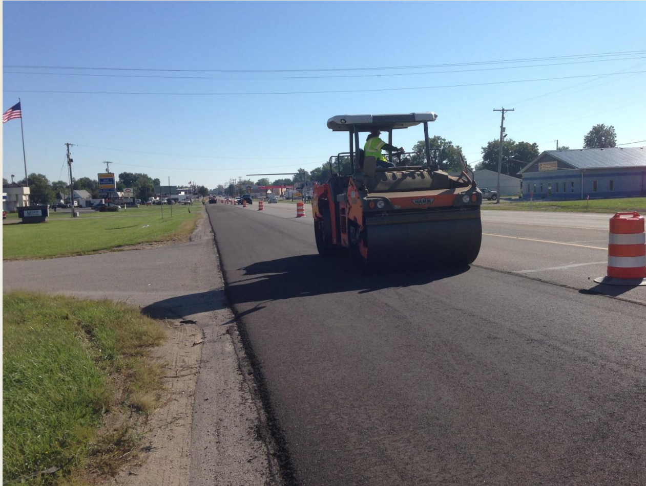
Compacting WB CIR 2014
