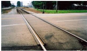
Rubber Seal and Asphalt
