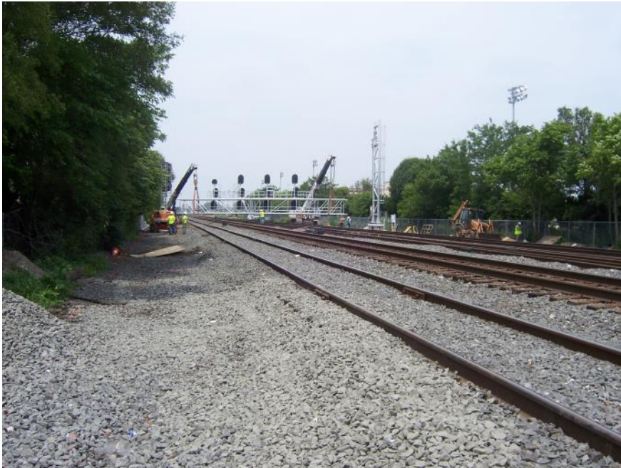
Setting the 4-track Signal Bridge
