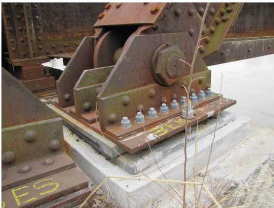
Replaced expansion bearing & pedestal
