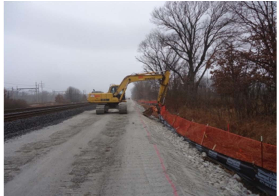
Compacting and Shaping Subballast
