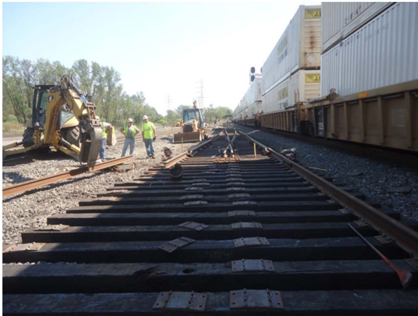
Assembling a new No. 20 Turnout
