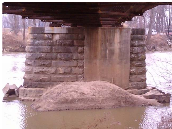
Replaced displaced masonry units with concrete facing
