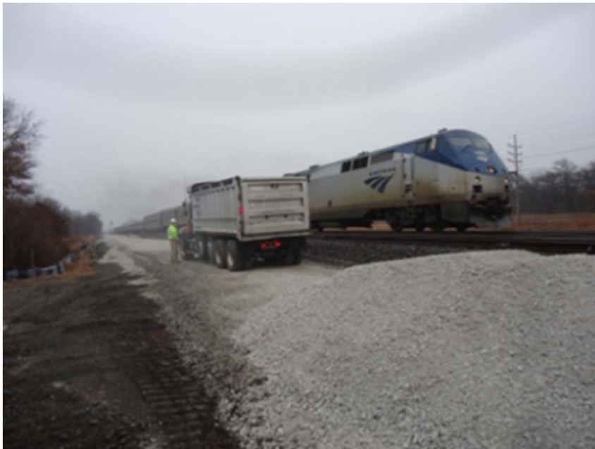
Delivering Subballast Stone
