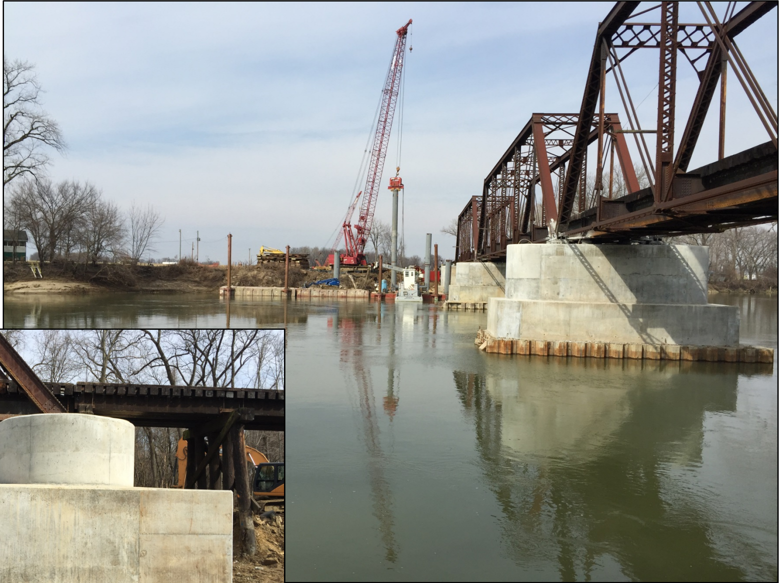
COMPLETED PIER RETRO-FIT
