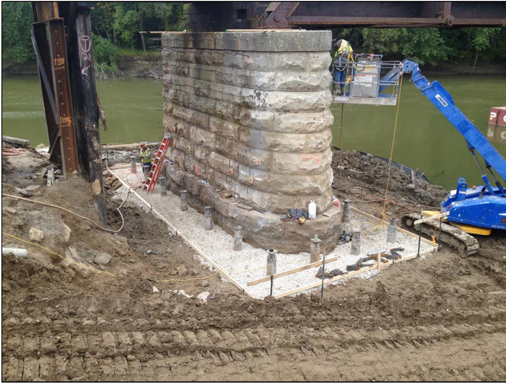
PIER 1 COMPLETED MICRO-PILE
