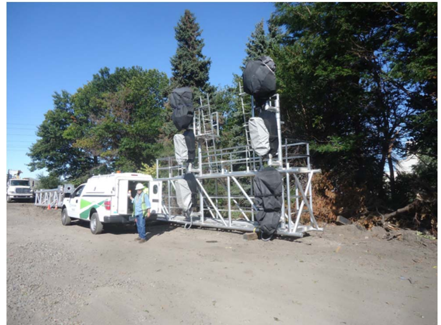
Preparing New Signals
