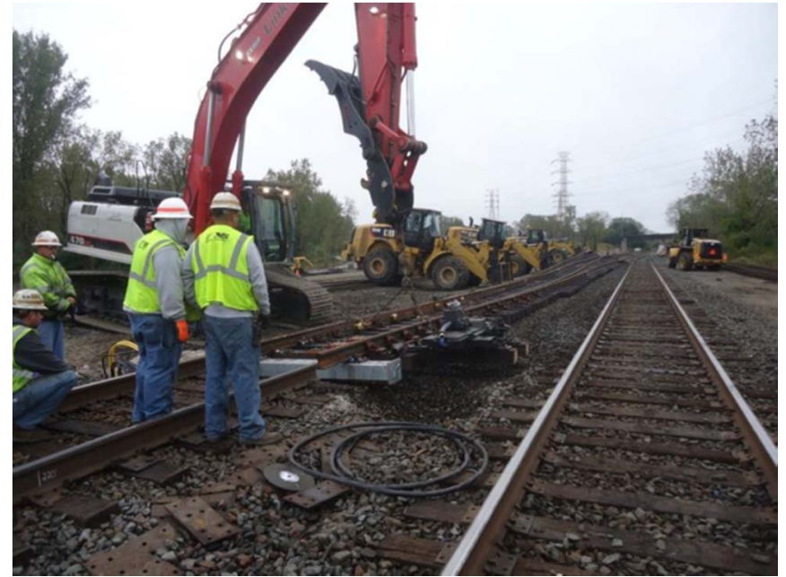
Installing a No. 20 Turnout
