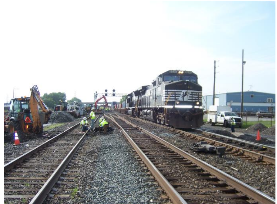
Track Construction on a Very Active Railroad
