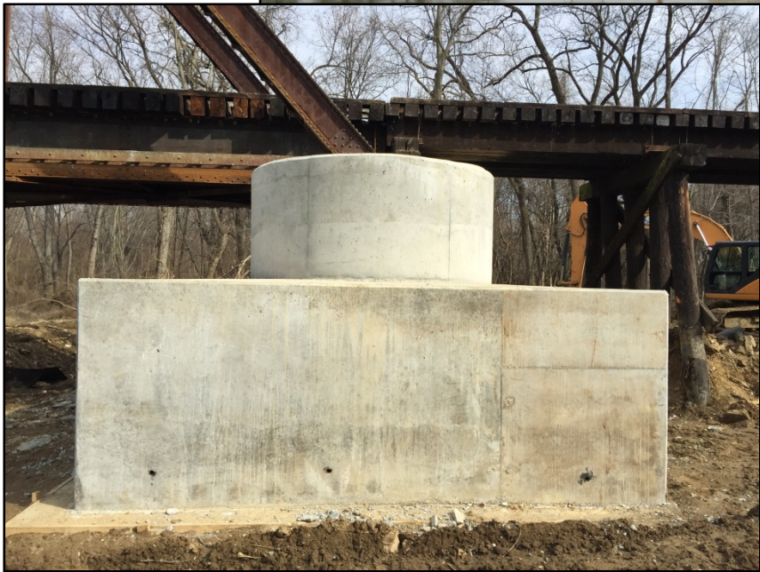
COMPLETED PIER RETRO-FIT
