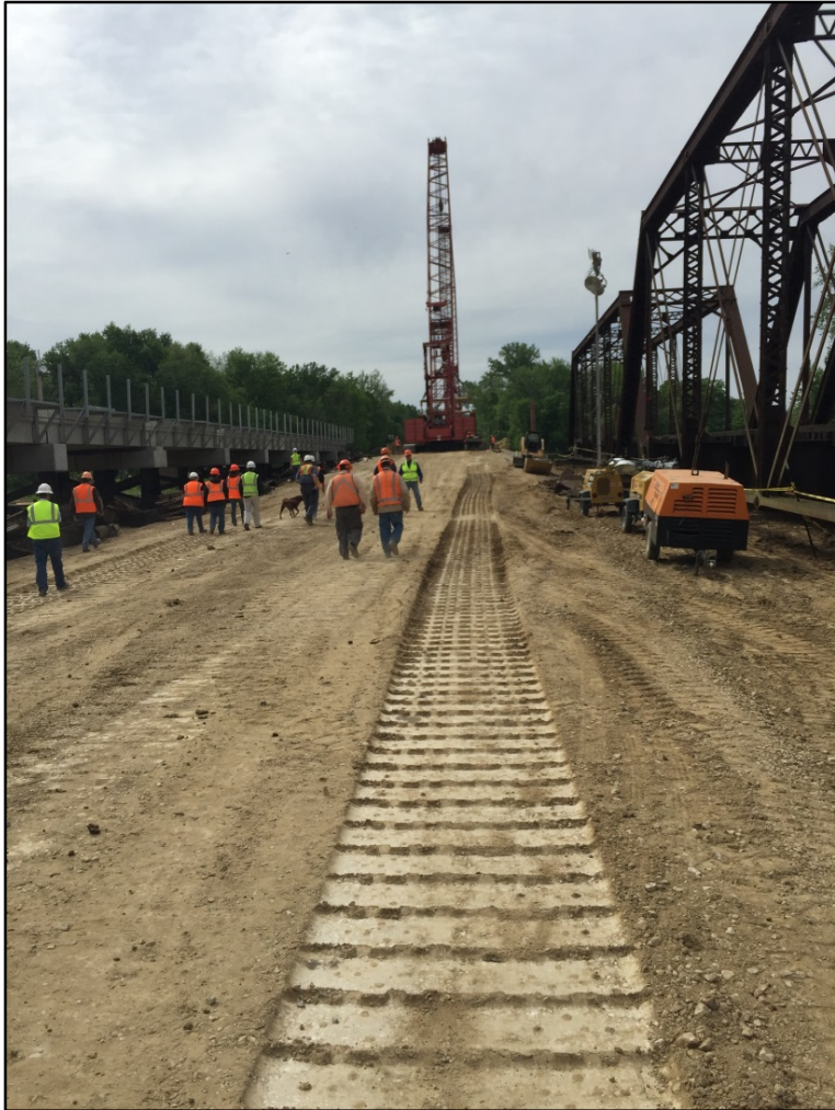
Main Span in transit. Note: 2" Depth tread marks from 500 kip load
