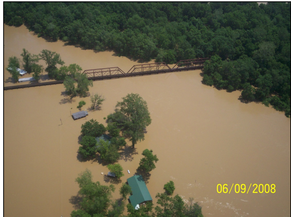
HAD TO CLOSELY MONITOR RIVER GAUGES TO MOVE EQUIPMENT AND MATERIAL BEFORE A FLOOD EVENT
