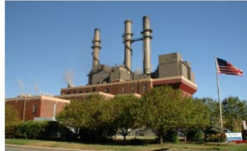
Citizens' Perry K Steam Plant utilizes clean-burning natural gas in its 8 boilers to generate 240°-600° F steam to heat buildings throughout the downtown area.
