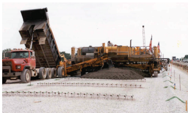
Figure 1 Typical PCCP paving.
