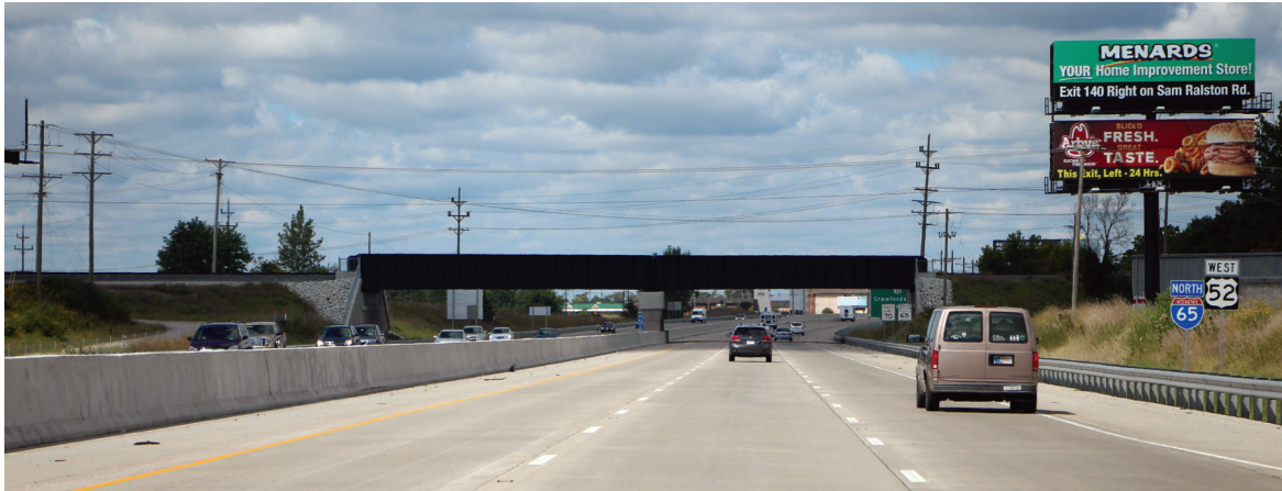
Figure 7. Construction zone on I-65 in Lebanon, Indiana.
