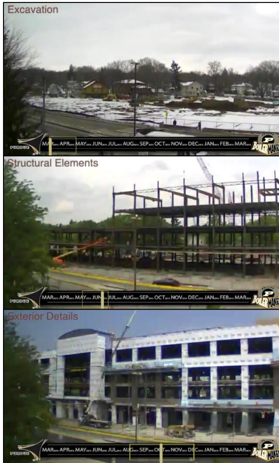
Wang Hall Construction, Purdue University
