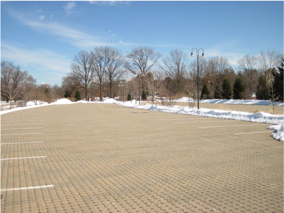
Figure 10.2.5 Example of Permeable Paver Parking Lot Installation at The Morton Arboretum, Lisle, IL
