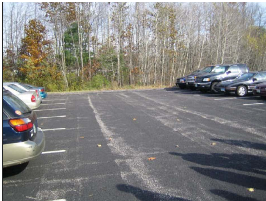
Figure 10.2.1 Example of a Porous Asphalt Parking Lot
