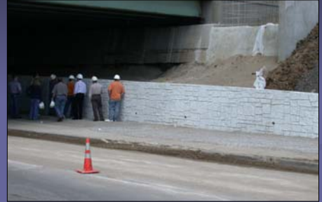
Retaining wall on 10 th Street for Monon Trail Extension
