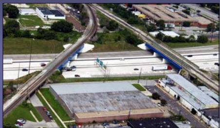
Bridge Painting / Masonry Coating
