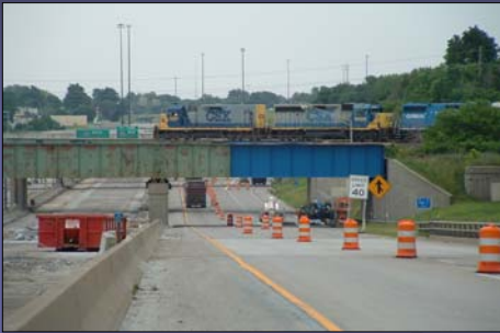
Railroad Bridge Painting
