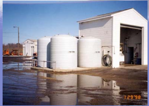
Traditional brine facility
