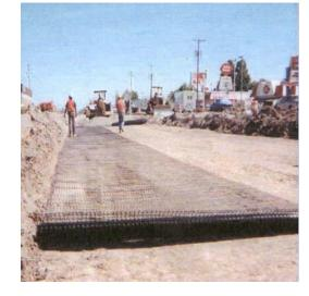
After encountering soft subgrade under the mainline and turn lanes, geogrid was installed after consultation with the INDOT Project Engineer.
