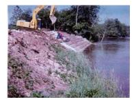
Geogrid combined with nonwoven geotextile in welded wire baskets and riprap fill. Terraced slope treatment used to restore and stabilize a breach in narrow bank separating the White River from an oxbow lake.
