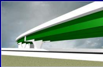
Steel Plate Girders With Integral Pier Caps
