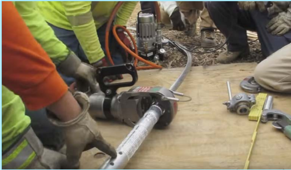
Figure 4 - Full tension ACSR splice installation with swage system
