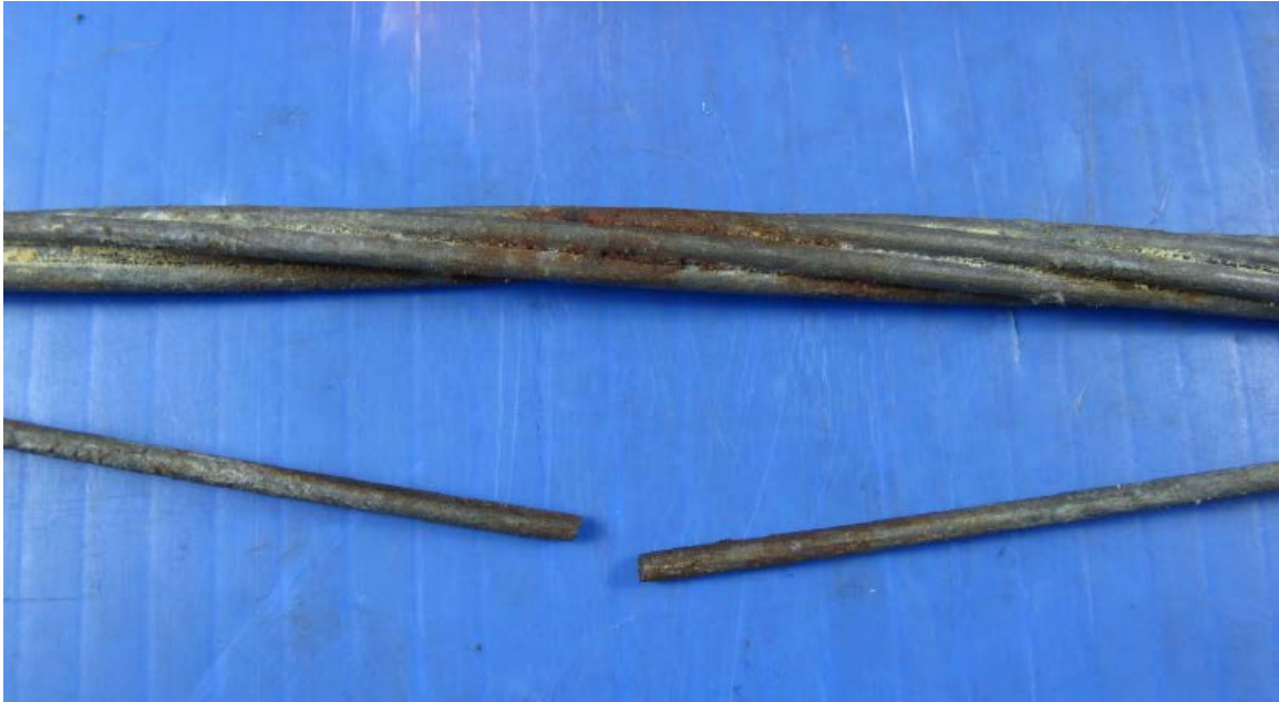
Figure 27 - L2312, Str. 39-40, Galvanized Steel Wires
