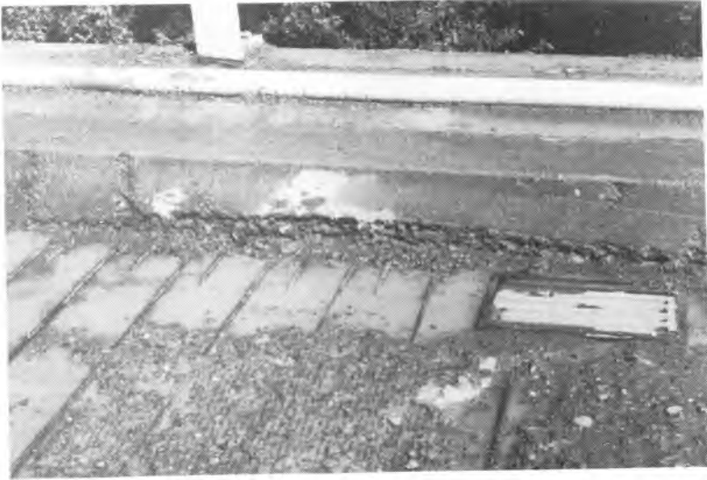
Finished curb section showing concrete surface for bonding and clean re-steel.
