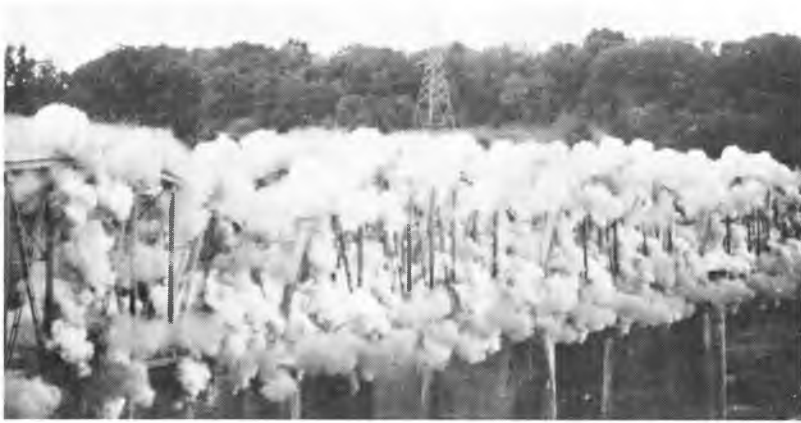
Figure 4. Photo of blast—smoke from primer chord and explosive charges.
