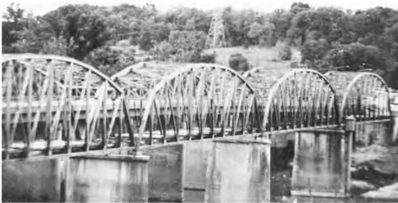
Figure 1. Existing Four Span Bridge
