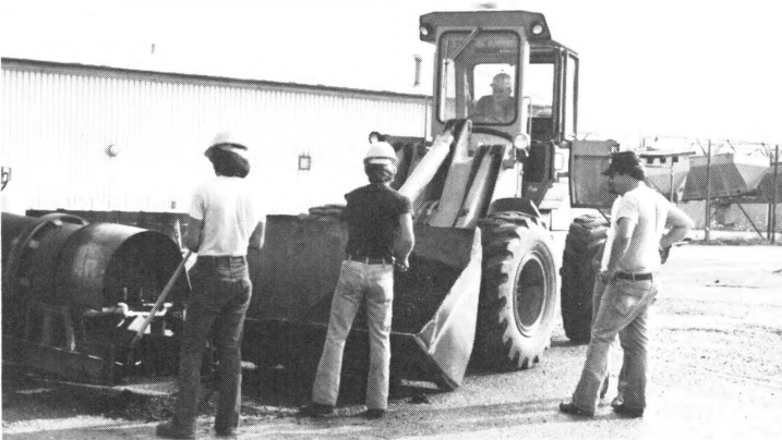
Figure 13. Heated Mix Coming Out.
