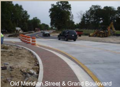
Old Meridian Street & Grand Boulevard
