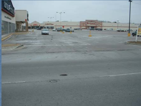
Kimco North Entrance facing East (Another view)
