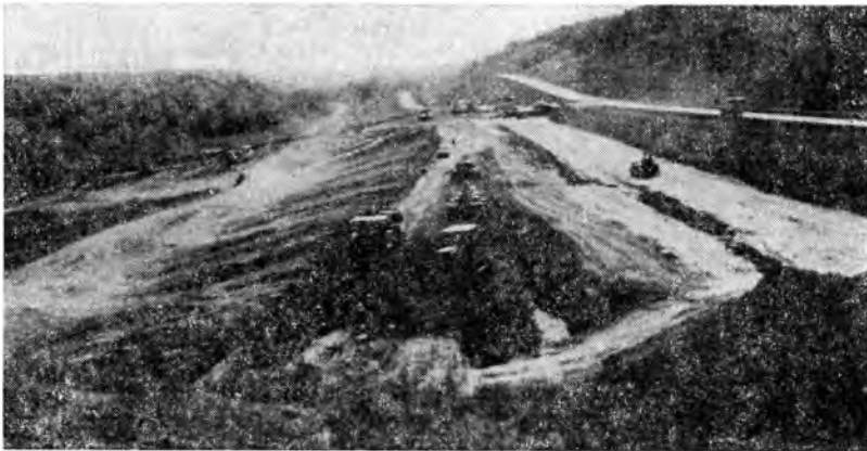
Photo 4. Embankment construction operations on I-74 River Slide.
