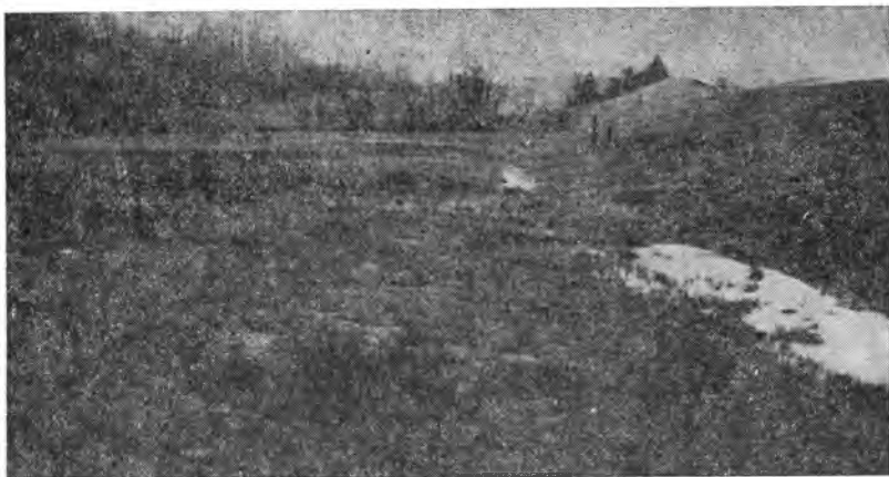
Photo 17. Completed landslide correction on I-74 Big Slide.
