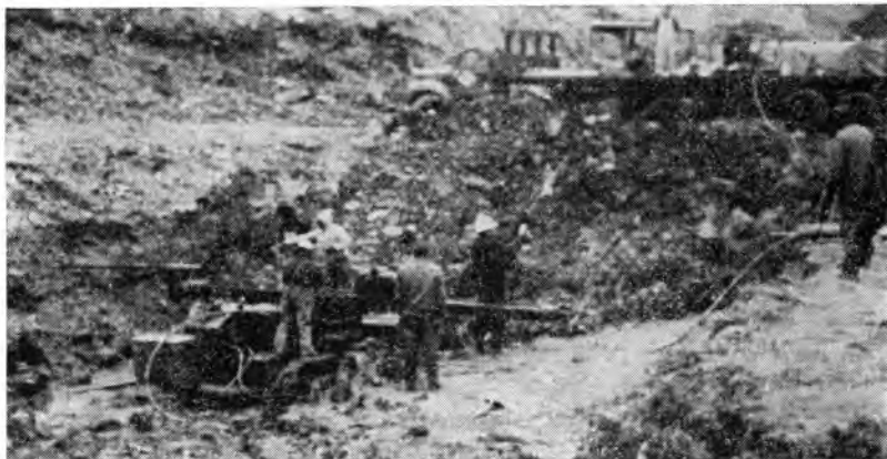
Photo 5. Horizontal drains being installed in I-74 Chicken Slide.
