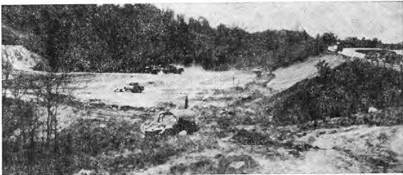
Photo 16. Construction of stabilizing berm on I-74 Big Slide.
