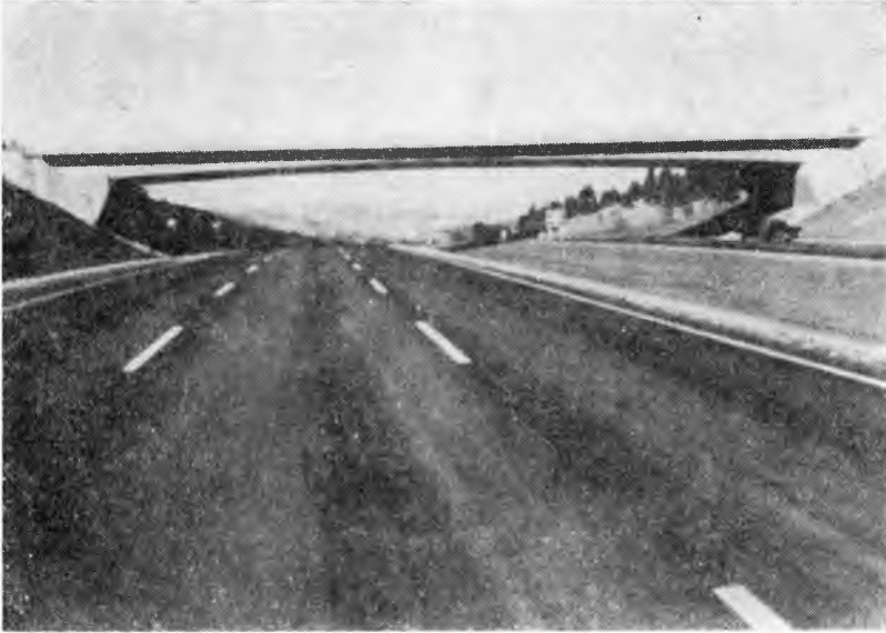
Fig. 1. No median pier collisions are possible at this Colorado bridge.
