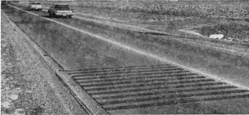
Fig. 1. Experimental Rumble Strips in Indiana.
