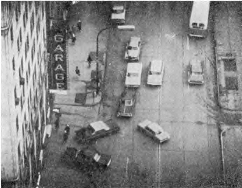
Fig. 4. Lack of auxiliary lane for left turning vehicle results in half the street being blocked.
