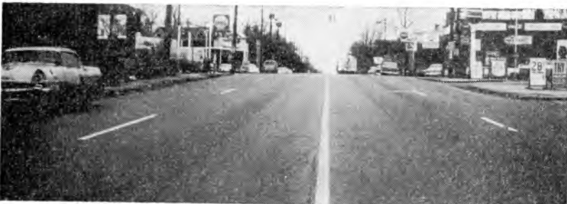
Fig. 6. Parking is prohibited on approach side and permitted on exit side. The cross street is one-way to the left, therefore, the curb lane has no place to go.
