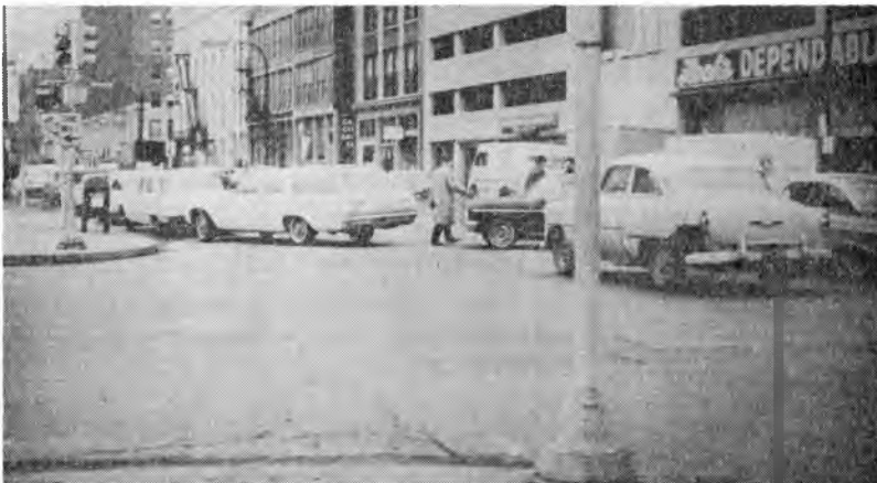
Fig. 2. Vehicles from cross street entering line to off-street facility blocking intersection.
