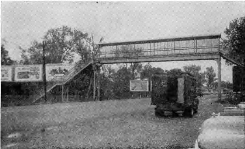
Fig. 13. Overpass school crossing at Evansville.
