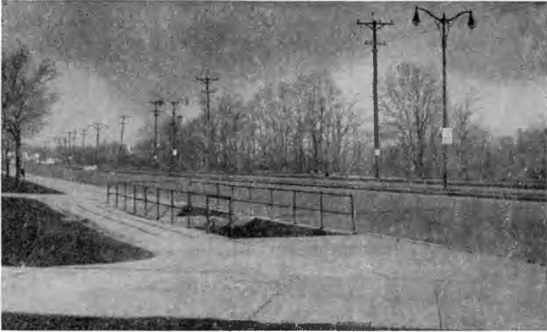
Fig. 12. Underpass school crossing at Richmond.
