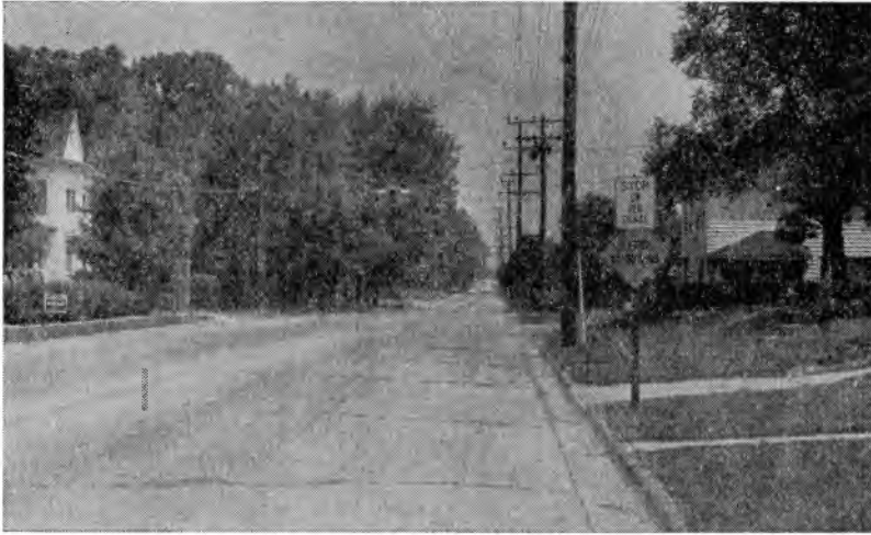
Fig. 8. Pedestrian-actuated signal installation at Lafayette.
