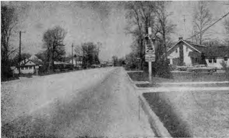
Fig. 6. Traffic control device used—special speed limit sign with horizontal alternate flashing signals.
