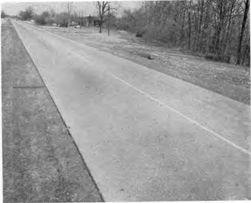
Fig. 1. Bituminous concrete overlay on State Road 37.
