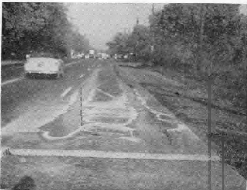
Fig. 8. Trench cut in bituminous overlay.
