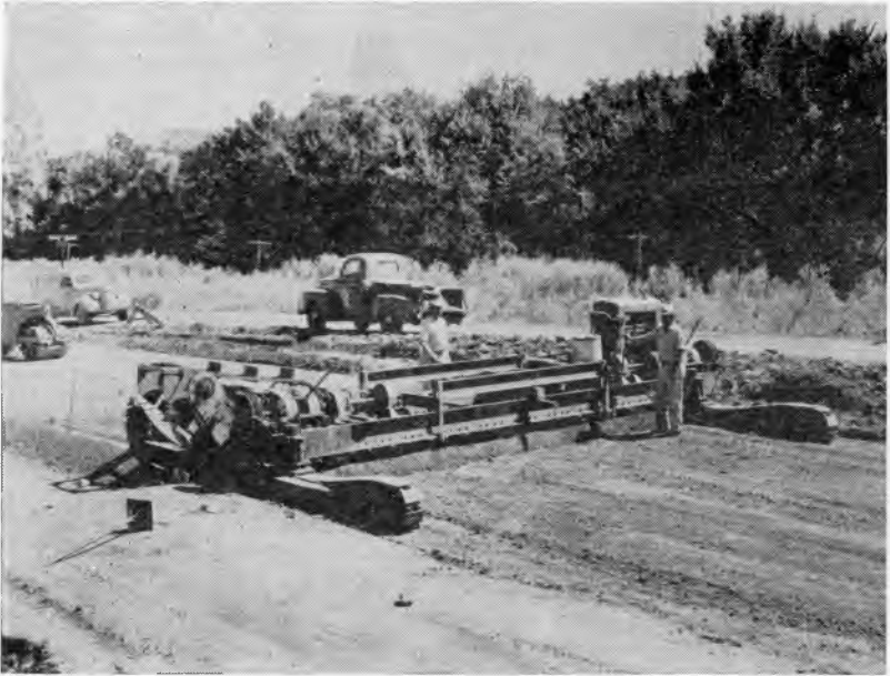
Fig. 11. Front view of another type of subgrader on which wheels were replaced with tracks and chain drives used to propel the machine.
