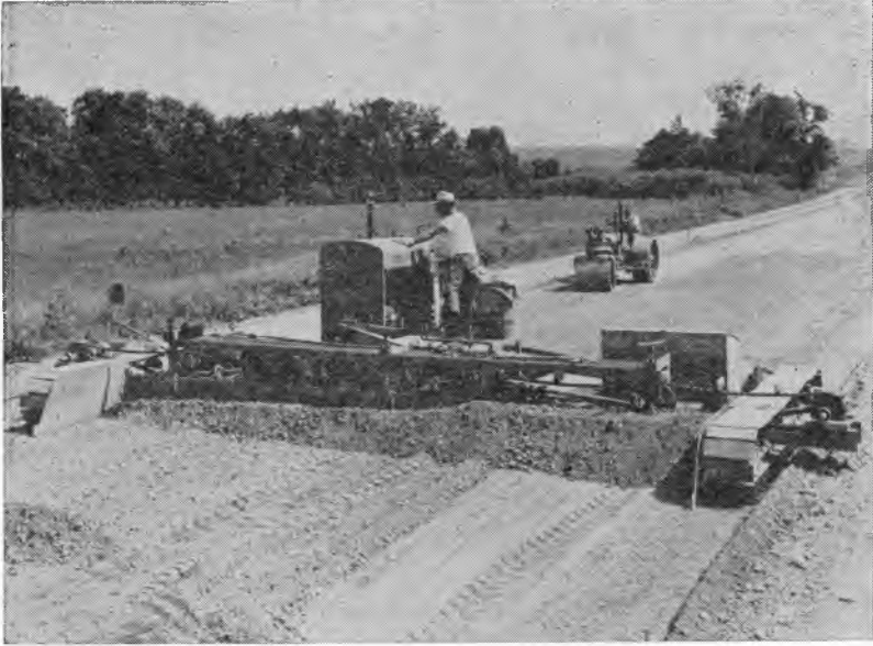
Fig. 8. Heavy duty self-propelled subgrade machine developed for constructing subgrade.
