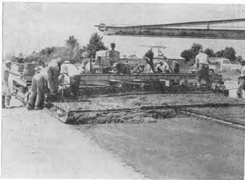
Fig. 5. First self-propelled machine designed to construct full-width course—front view.
