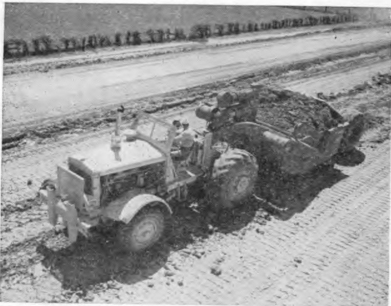
Fig. 4. An earth mover places a six-inch lift of soil on one of the AASHO Road Test loops. The A6 type soil was then bladed, mixed, and compacted. Specifications called for density to be controlled between 95 and 100 per cent of standard maximum, and moisture content between plus or minus two per cent of optimum.
