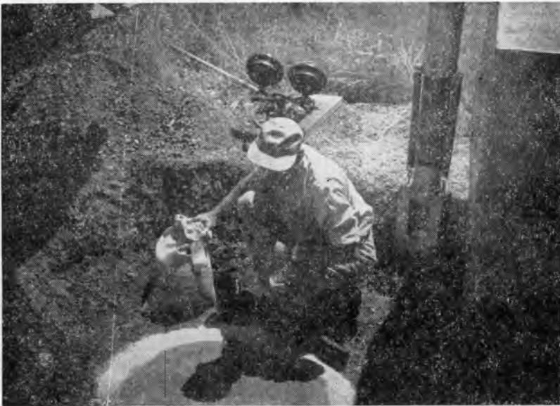
Fig. 2. Placing sand layer on base in preparation to seating the plate.
