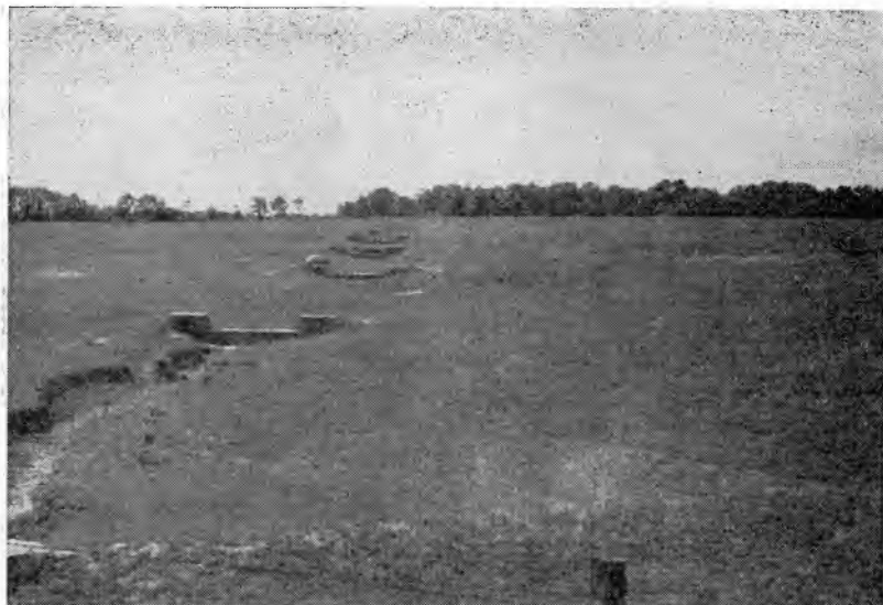
Fig. 16. Check dams to retard erosion in Illinoisian Drift area of Decatur County, Indiana.
