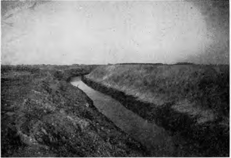
Fig. 18. Ditch practice required to drain Wisconsin Drift area in White County, Indiana.
