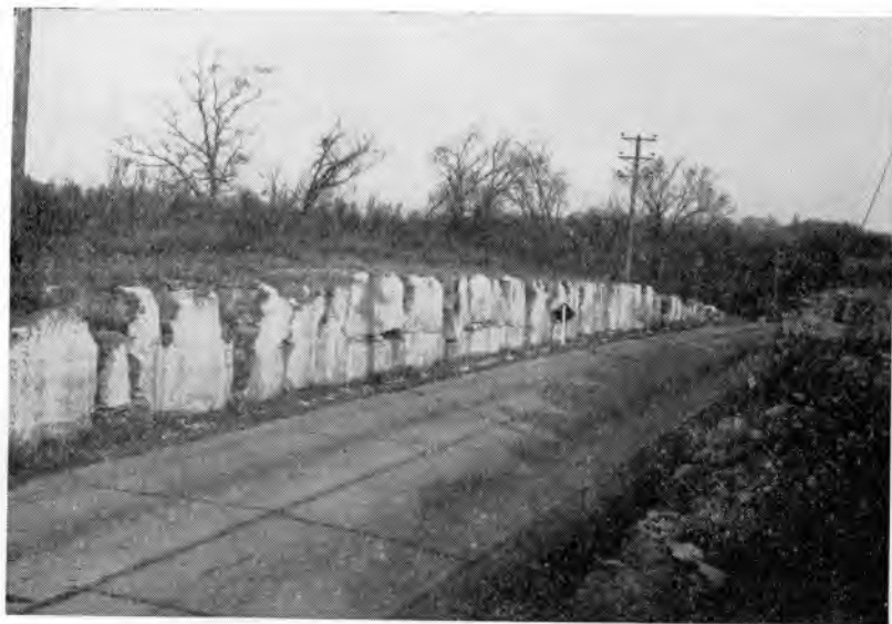
Fig. 8. Highway excavation in Mississippian Bedrock (L.S.) near Bedford, Indiana.
