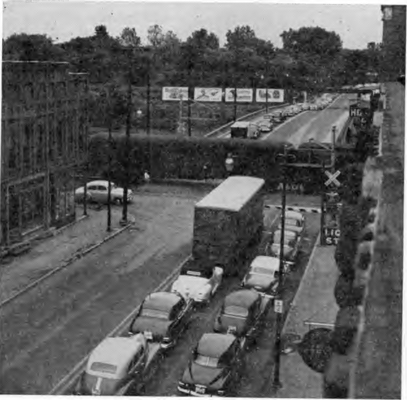
Fig. 22. This view illustrates the costly delays which occur frequently at railroad grade crossings. Traffic problems such as this are being studied by the Joint Highway Research Project in several Indiana cities. (30219)
