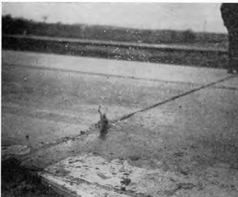
Fig. 5. This view shows a "water squirt"—a new and serious highway problem known as "pavement pumping." (4713)
