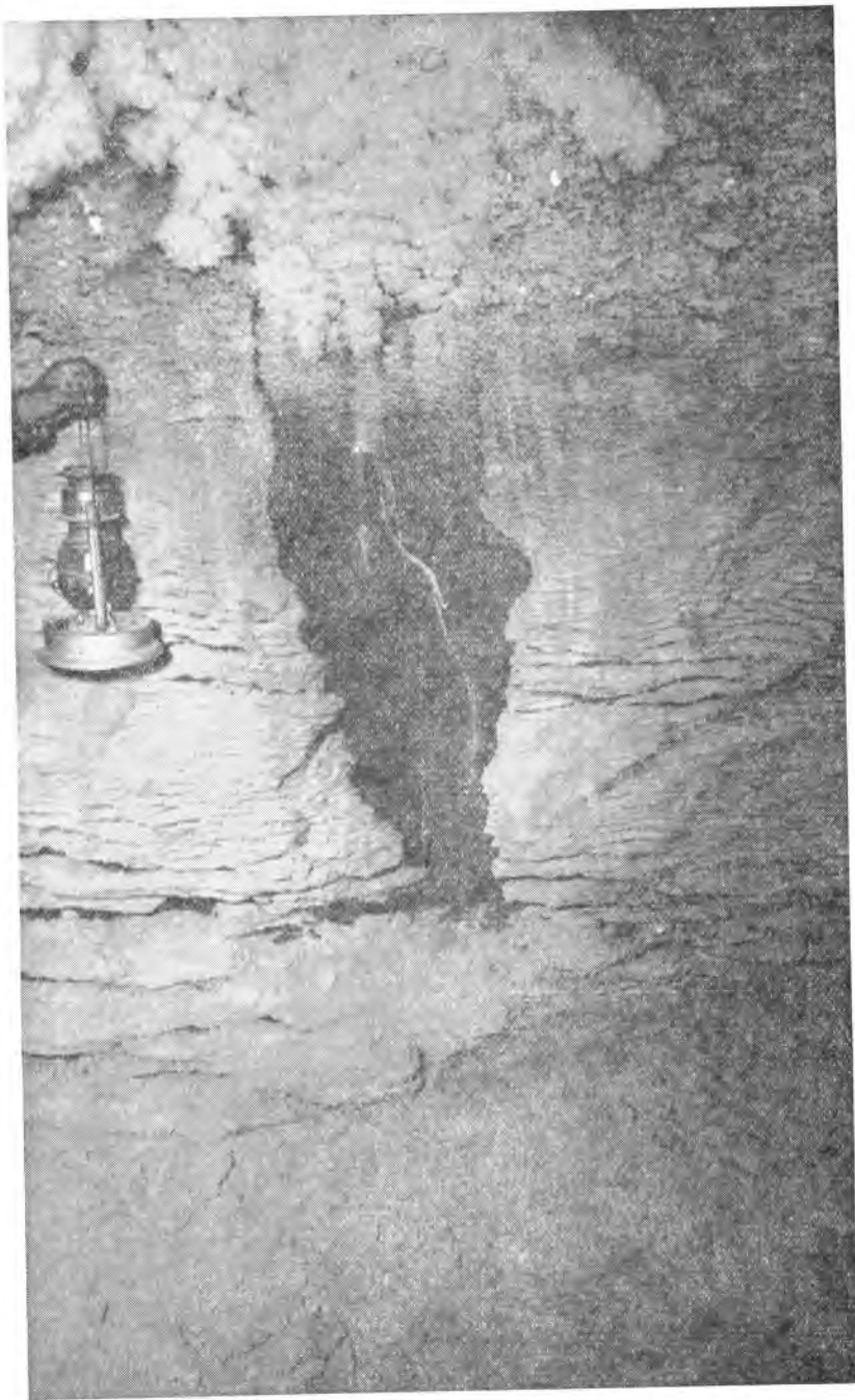
FIGURE 3. Ice Wedge in a Cold Storage Cave. This wedge extends downward at least 20 feet below the surface. Note the horizontal sills of ice. The frost accumulation on the upper part of the walls and on the ceiling is frozen vapor from the workmen's breath.
