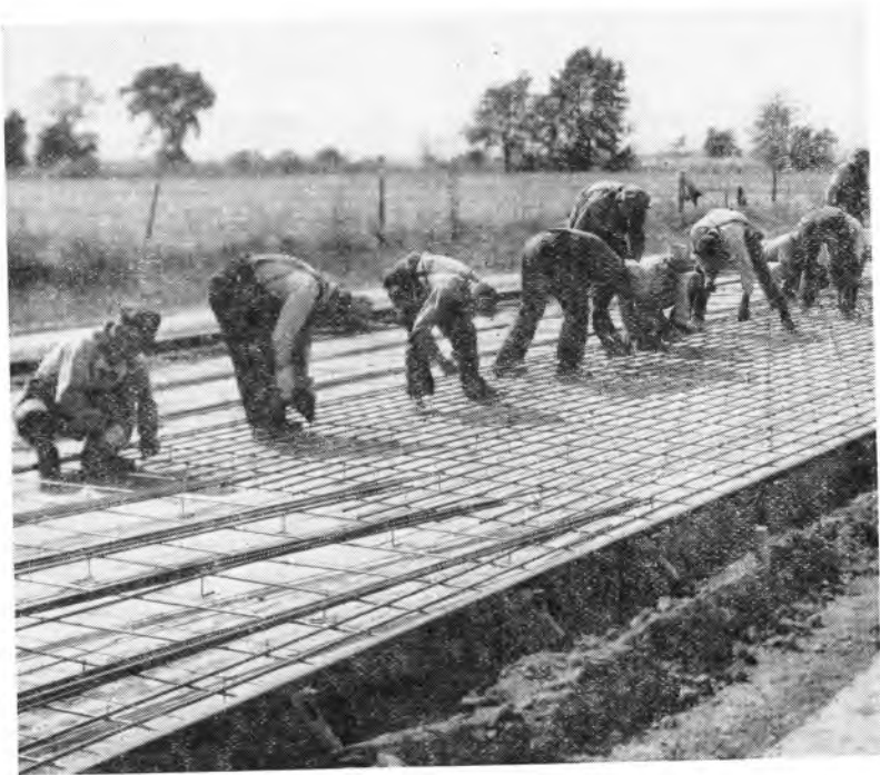
FIGURE 1. Workmen placing and tying longitudinal steel for experimental pavement.
