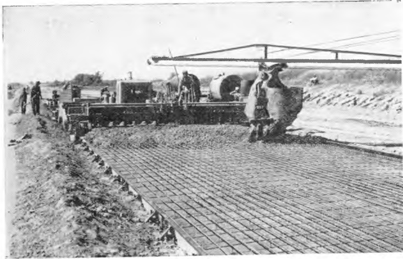
FIGURE 3. Placing concrete on continuous reinforcement.
