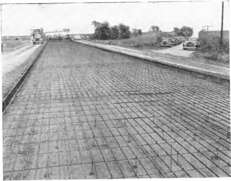
FIGURE 2. Complete assembled continuous reinforcement.
