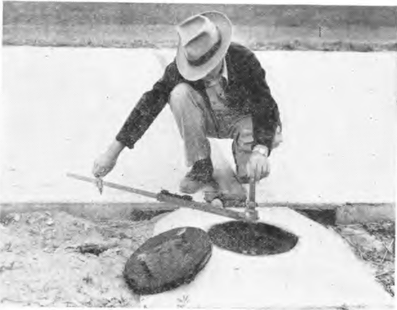
FIGURE 4. Measuring horizontal and vertical movements from a reference monument.
