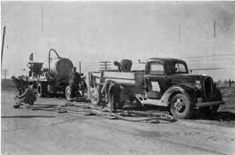
Mud-jack crew filling voids under concrete pavement.
