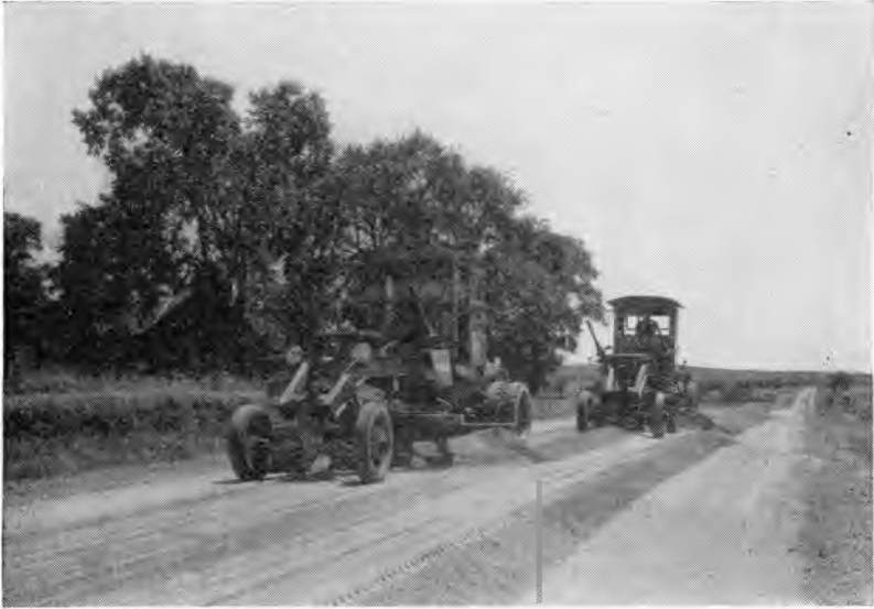
Drying aggregate before applying bituminous material.
