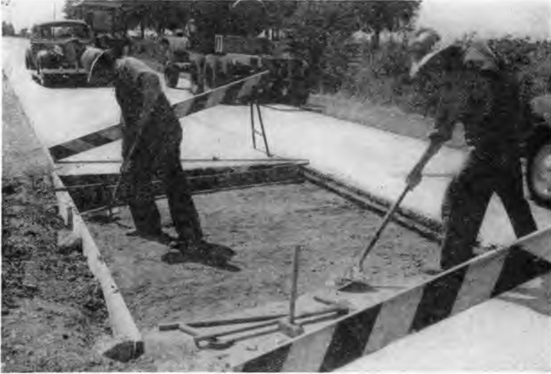
Preparing subgrade to receive concrete patch.
