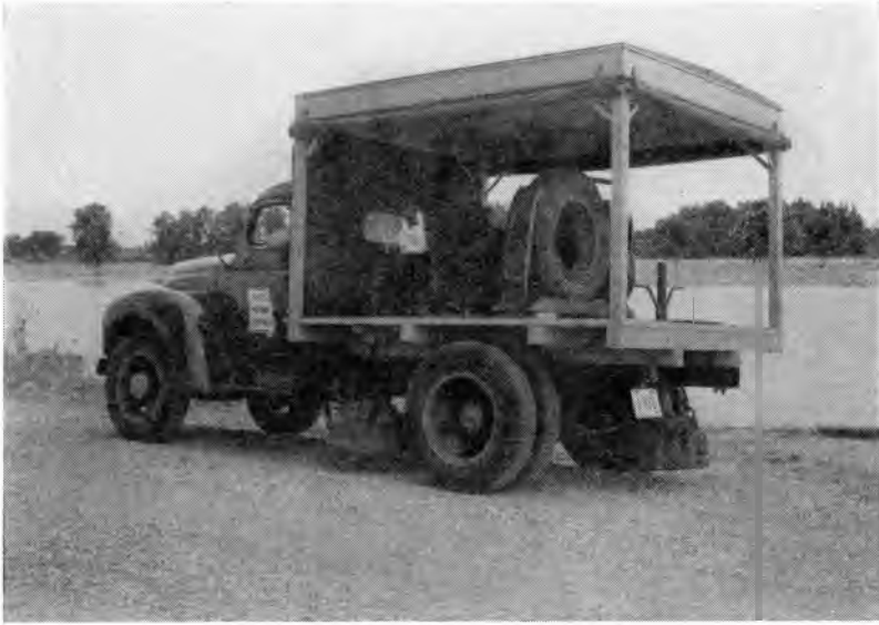
Road magnet used to remove pieces of metal from road surface.
