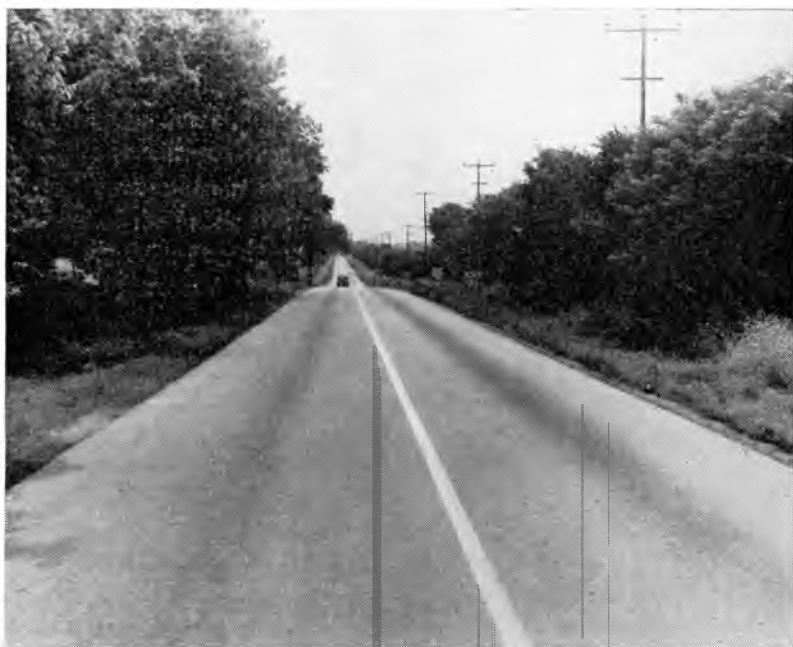
Excellent performance of plant-mix bituminous surface on U. S. 60 near Versailles. The application was about 75 pounds laid over an existing bituminous pavement. Construction—1943; traffic—approximately 5,000 vehicles per day, 1,250 of which are trucks.
