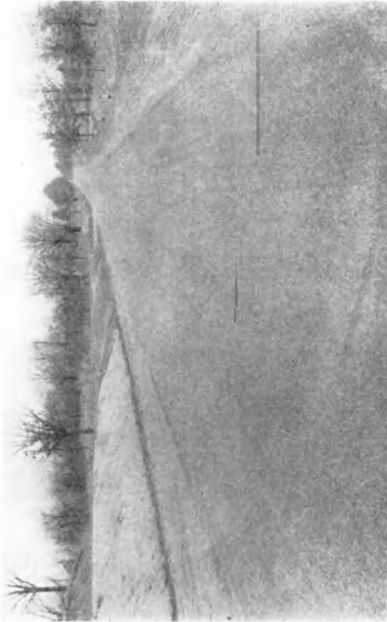
Fig. 4. An example of good performance of a flexible pavement on granular soil (Bellefontaine).
