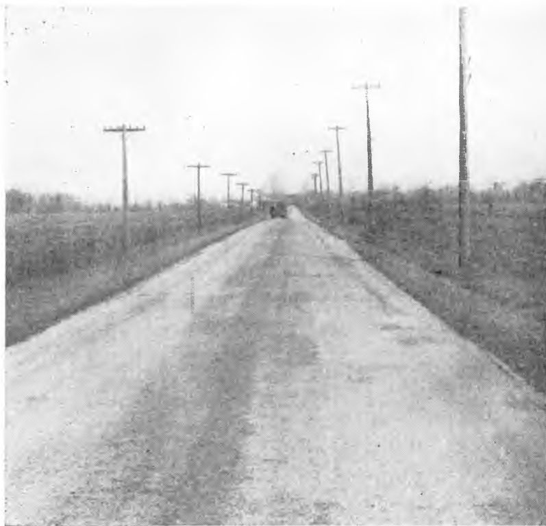
Fig. 3. Good performance of a flexible pavement placed on granular soil (Fox).
