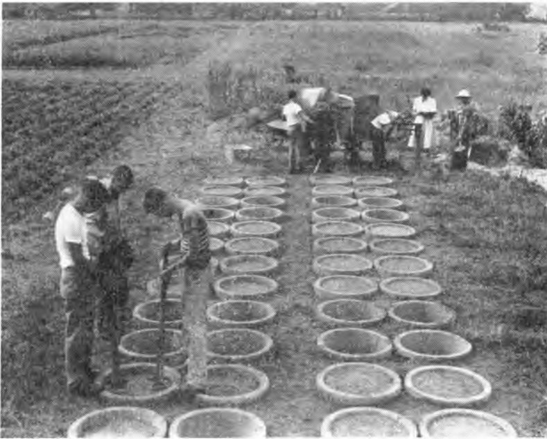
Fig. 3. View of the experiment where various mixtures of aggregate materials are being installed to study the factors influencing establishment of turf. Note that the materials were weighed, mixtures were prepared with a power mixer, and mixtures were compacted by hand tamping.
