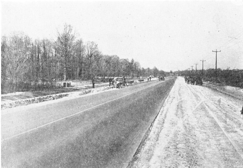
Fig. 3. Widening shoulders after pavement widening on U. S. 31 south of Scottsburg.
