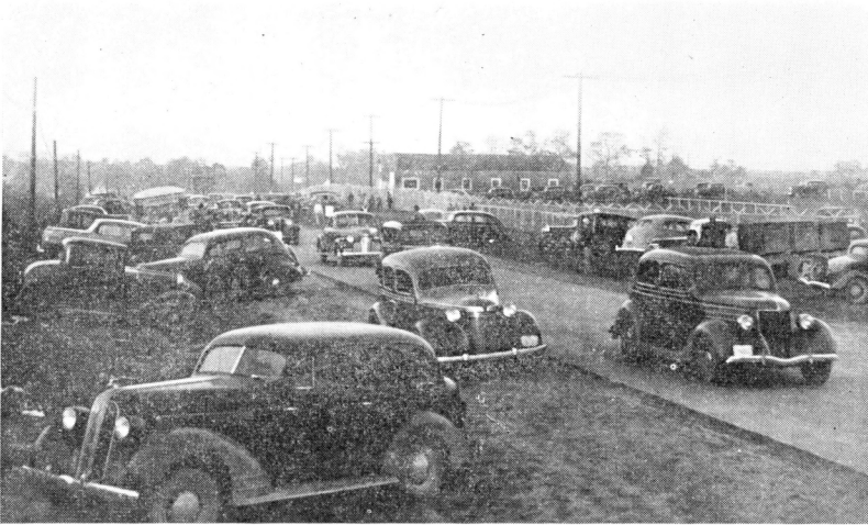
Fig. 4. Traffic confusion on State Road 62 at Charlestown Powder Plant before dual-lane construction and addition of pedestrian overhead structure.
