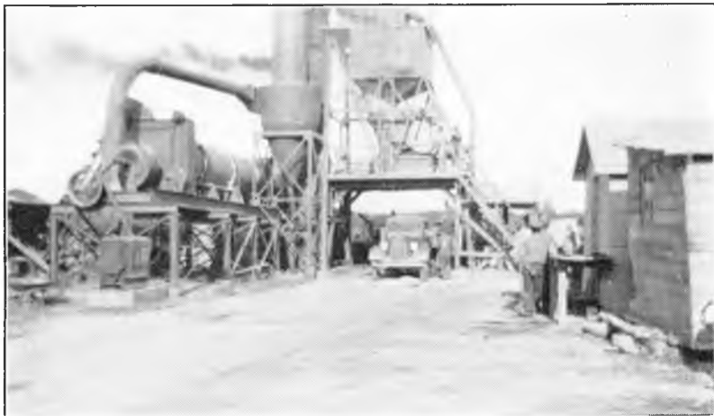
Fig. 2. A modern portable asphalt plant of one-ton mixer capacity.
