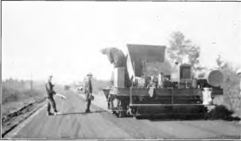
Fig. 4. View of mechanical spreader on two-layer, part-width operation.
