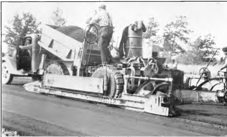
Fig. 3. A mechanical spreader for two-layer, part-width spreading of oil aggregate.
