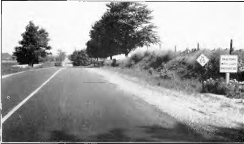
Fig. 1. A plant-mix, oil-aggregate surface on M - 66 near Six Lakes.
