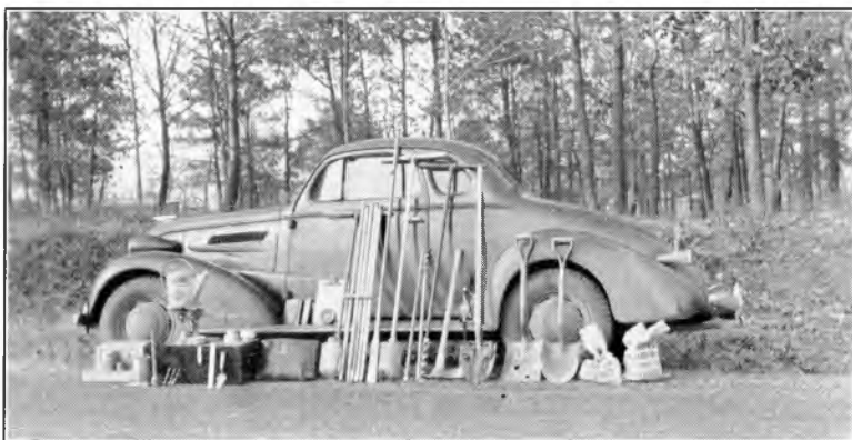
Fig. 3. Field equipment used in obtaining soil profiles by the Bureau of Tests, Ohio Department of Highways.
