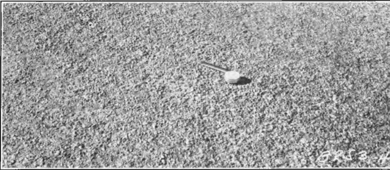
Fig. 9. A typical non-skid surface as developed by the California State Highway Department. Hot 94 + road oil covered with \frac{1}{4} -inch to \frac{1}{8} inch screenings. The use of screenings of this size makes an effective non-skid cover which will not be kicked out readily by traffic.
