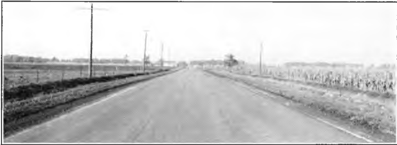
Fig. 7. General view (1936) of sandstone rock asphalt, A-2 type (see Fig. 3), on Indiana State Road 29 between Burlington and intersection with State Road 28. Rock asphalt surface treatment placed on an old penetration macadam in heated condition in June, 1936. The surface was smooth and had a typical "sandpaper" finish similar to the rock asphalt surface tested in the 1933 skid tests.
