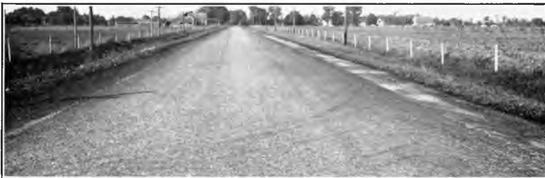
Fig. 5. General view (1936) of penetration macadam, A-5 type (see Fig. 3), on Indiana State Road 29 between Deer Creek and Burlington. A penetration macadam surface treated in 1934 with a seal coat and an excess of cover stone \frac{1}{4} - to \frac{3}{4} -inch size, providing a rough open-textured type of surface. The cover stone was a fairly soft limestone with no oil showing on the exposed side. The sharp edges were worn smooth at the time of test. The surface was smooth riding, but the rough open texture caused a rumbling noise typical of this type of treatment.
