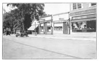
Fig. 2. State Route 55 through Crown Point. Same view as Fig. 1 after paving with reinforced concrete using combination curb and gutter.
