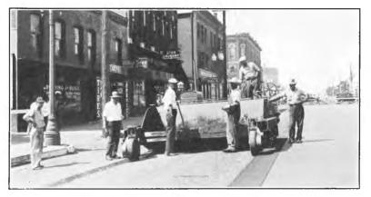
Fig. 6. U. S. Route 12 through Michigan City. Placing rock asphalt on binder course with an Adnun Finishing Machine. The three stages of the resurfacing work are clearly shown.
