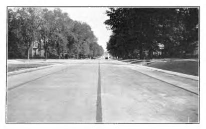
Fig. 4. State Route 55 through Crown Point. Looking southward from station 22+00 after removal of car tracks and construction of 36-foot reinforced concrete pavement.
