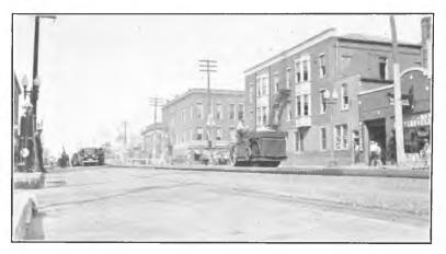
Fig. 5. U. S. Route 12 through Michigan City. Resurfacing old brick pavement with a binder course of asphaltic concrete and a wearing course of rock asphalt.
