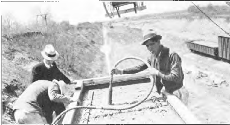
Fig. 4. Placing concrete in a structure by internal vibration.
