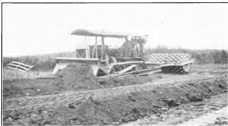
Fig. 1. Compacting subgrade with Sheepsfoot roller.
