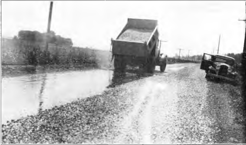
Fig. 1. Covering stone being applied from dump truck backing over fresh application of bituminous material.
