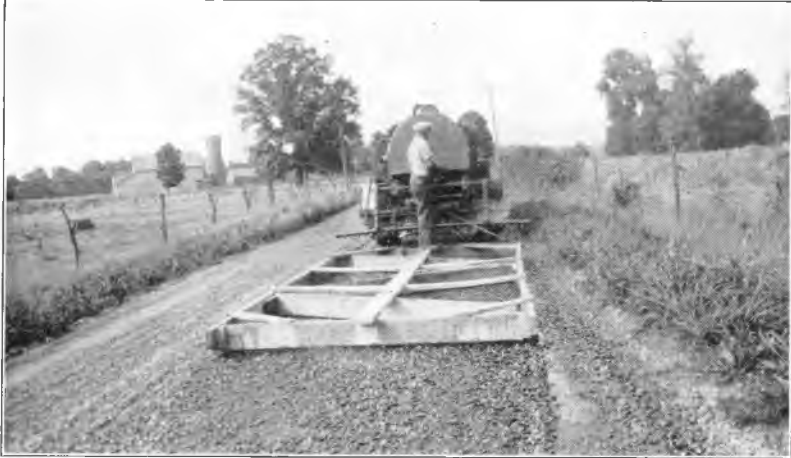
Fig. 2. Home-made wooden drag pulled by a distributor on county road surface treatment.
