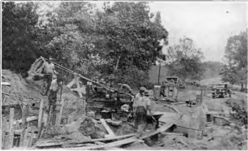
Fig. 2. Construction progress. Pump dewatering cofferdam for approach wall.
